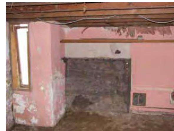
North interior elevation of room #4 with finishes and floor removed.
