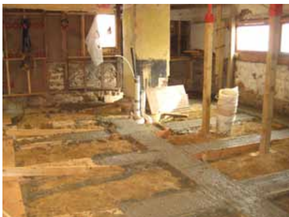
After concrete has been poured
