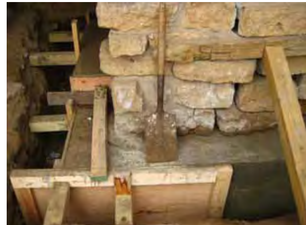
Underpinning at the stone foundation under Mr. Wright's Bedroom.
