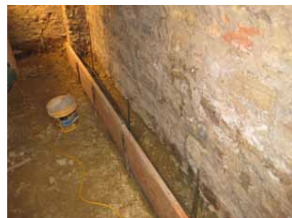
Trench in the boiler room ready for concrete to be poured.
